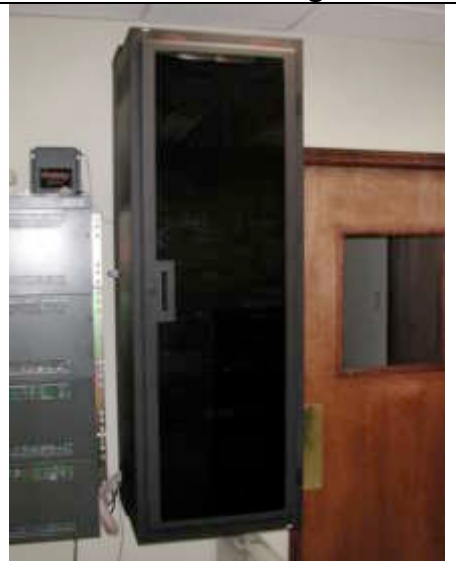
Figure 3.4 Cabinet housing firewall
